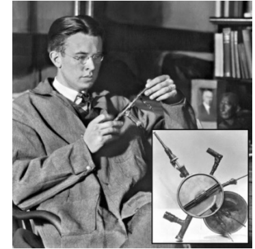
1930 E.O. Lawrence & M.S. Livingston – 80 keV cyclotron
